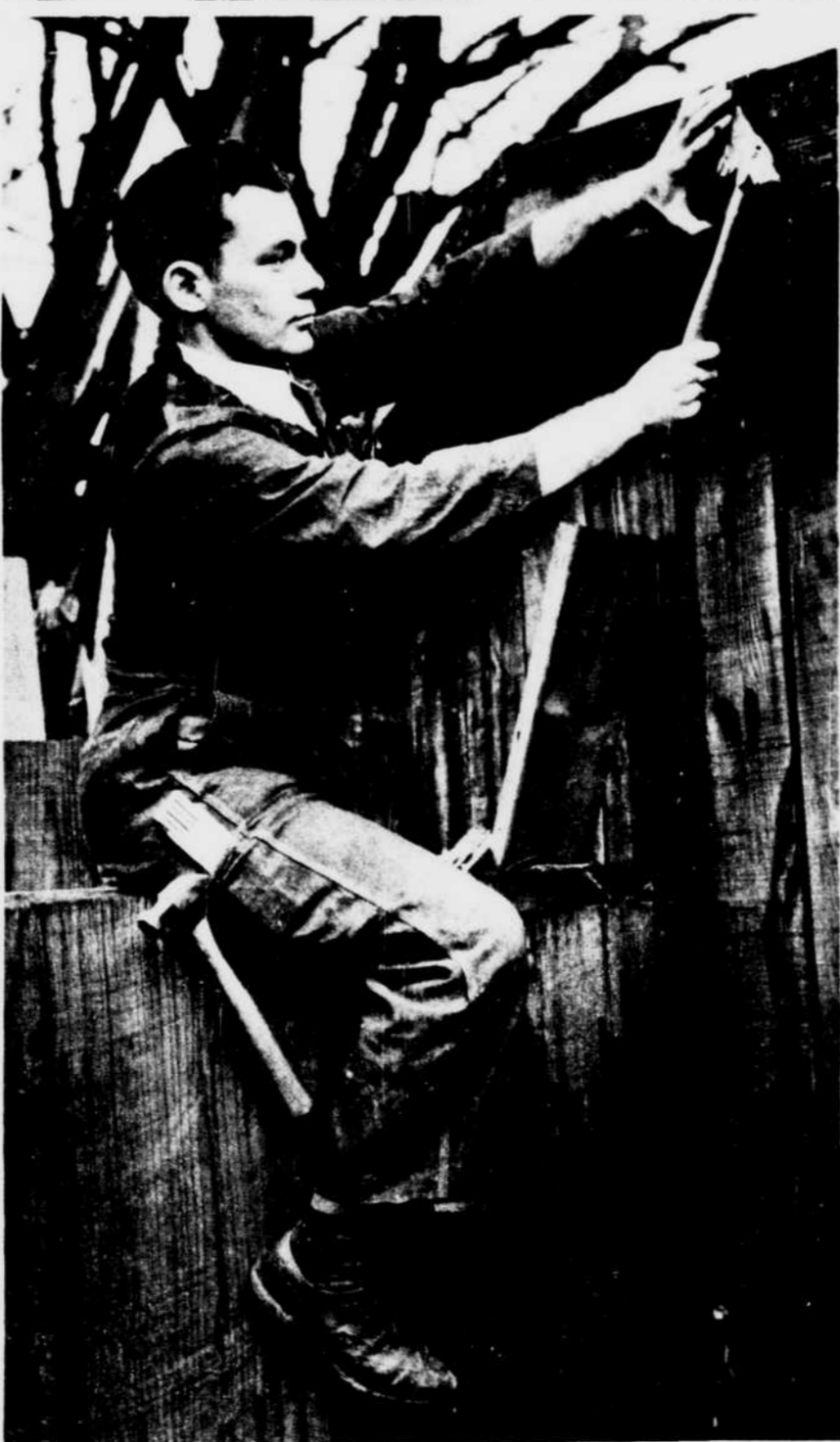
Repairing a dilapidated shed in the colored section of town is sturdy David Dobree. A dusty job, but it brings in as much money as violin teaching.
