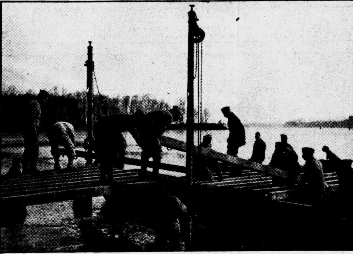
ARMY ENGINEERS TOIL—This is work more suited for summer, but Reserve officers taking the Army's engineering course at Fort Belvoir, Va., turn out in all kinds of weather. Here a group of them lay a pontoon bridge. That officer in the water is not wading without his shoes—he's wearing hip boots.
