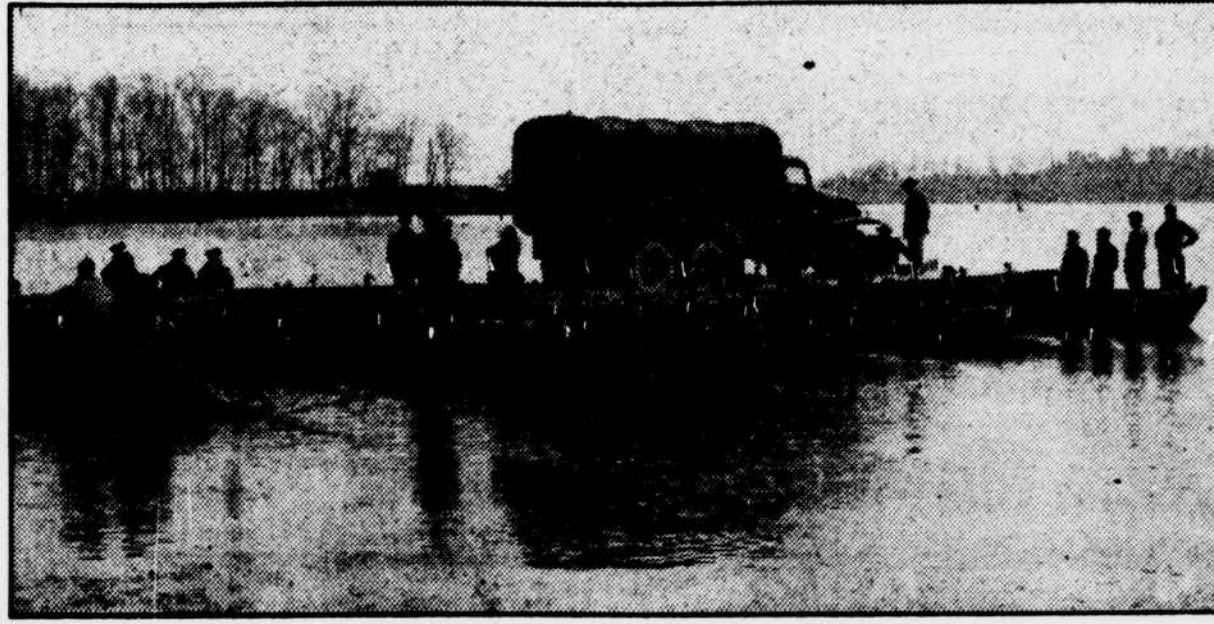
It works—that is the thrill Army Reservists get when they find their handiwork does its duty. A 10-ton truck has been moved out on a section of a pontoon bridge to test its strength. Regulars call the Fort Belvoir session a "refresher" course. The present course will end March 1 for the 200 Reservists.
