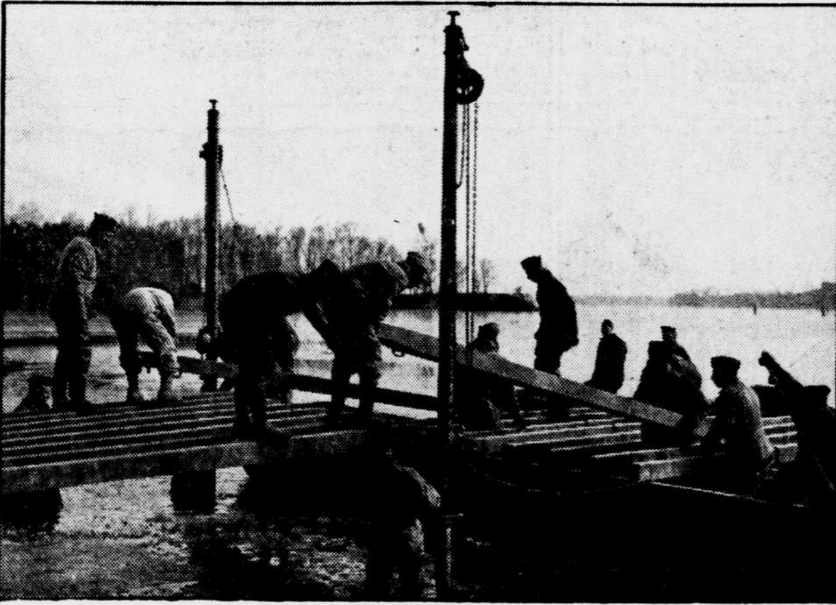
ARMY ENGINEERS TOIL —This is work more suited for summer, but Reserve officers taking the Army's engineering course at Fort Belvoir, Va., turn out in all kinds of weather. Here a group of them lay a pontoon bridge. That officer in the water is not wading without his shoes—he's wearing hip boots.
