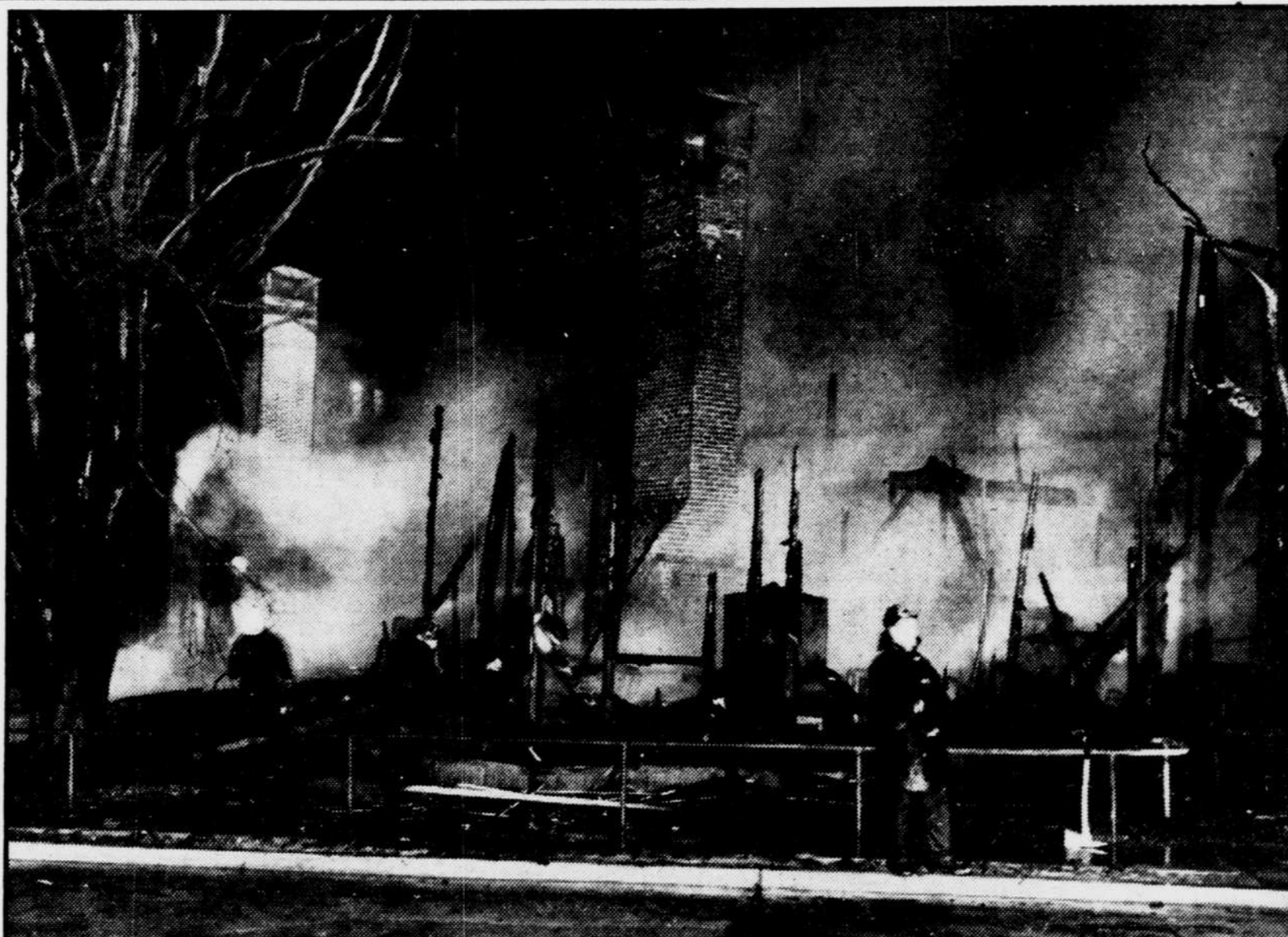
EARLY MORNING FIRE AT ST. ELIZABETH'S —Naked chimneys are all that remain of the two-story frame building, housing the St. Elizabeth's Hospital Red Cross recreation building, which was razed by fire early today. No one was reported injured. The building burned quickly and threatened empty Hitchcock Hall adjacent to it, until a large force of firemen managed to confine the flames to the Red Cross building. Damage was estimated at more than $15,000. —Star Staff Photo.
