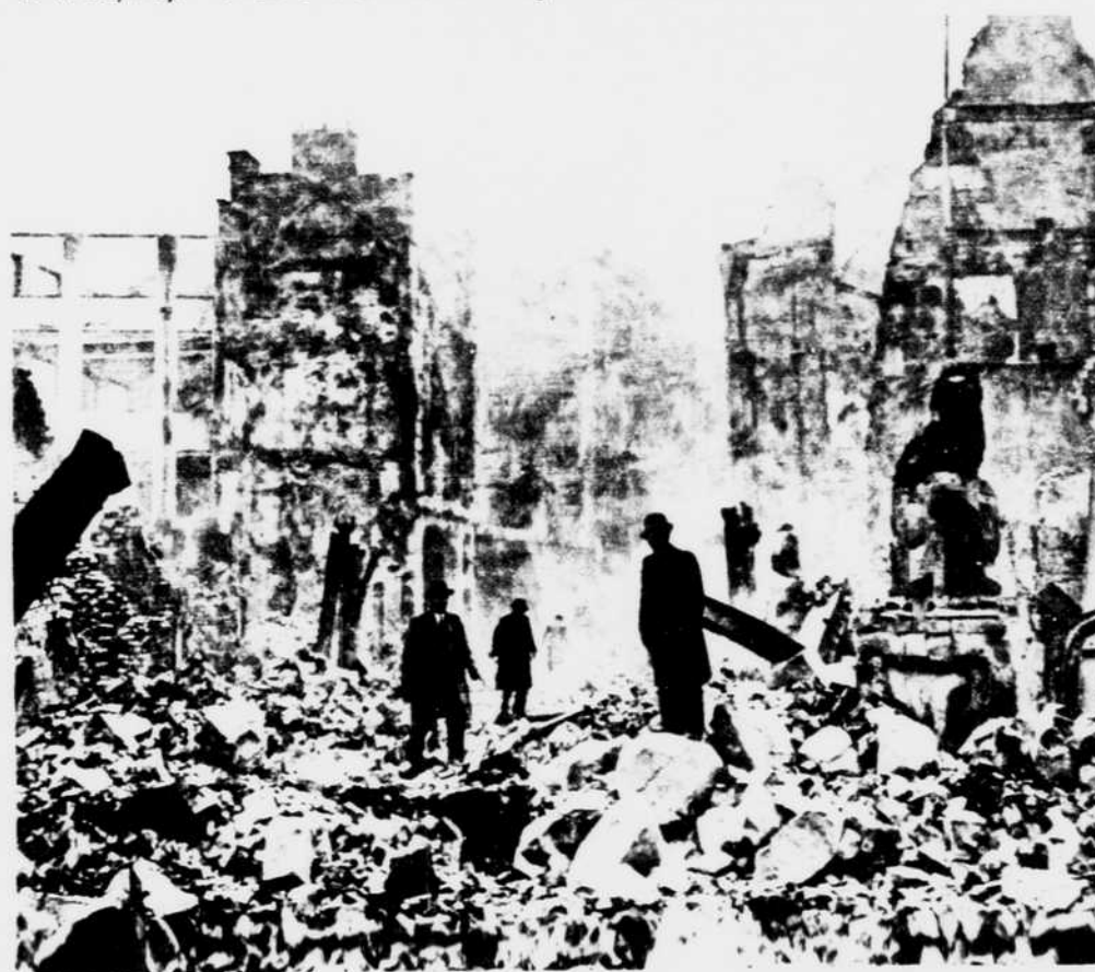
Shattered, smoke-blackened walls give the aspect of an architectural cemetery to this wrecked section of the ancient "City," rich in association with some of the most famous men and events in English history. Wide World and A. P. Photos.
