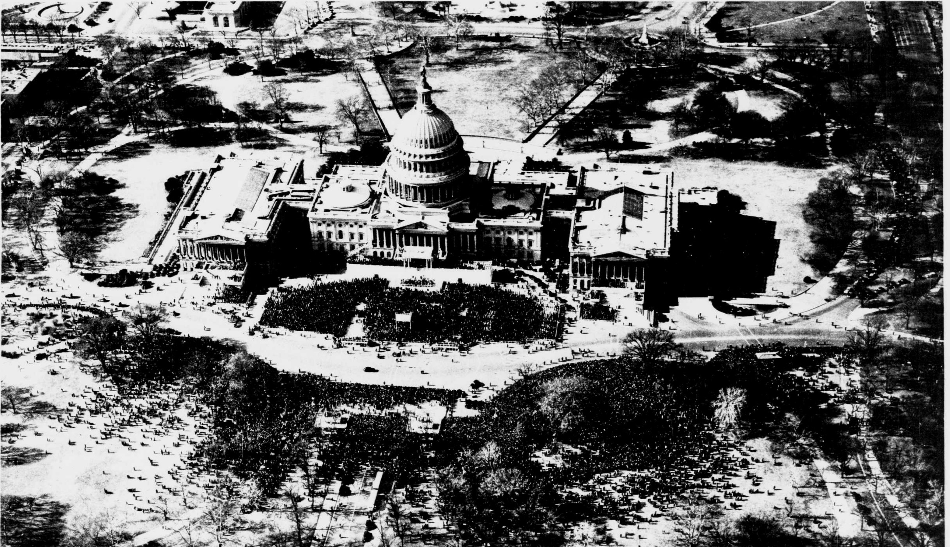
From the air above Washington, where this picture was made, the thousands who crowded around the Capitol and along the parade route looked like a bee swarm. Those who did not have tickets for the stands in front of
